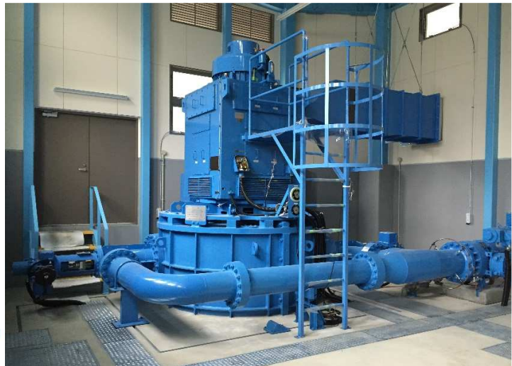
Figure 24 : Makayabaru turbine (Japan) designed from Mhylab's systemization ( Q_n = 0.5 \text{ m}^3/\text{s} , H_n = 181 \text{ m} , P_m = 800 \text{ kW} , 2 nozzles, 600 rpm) (© Nippon Koei)
