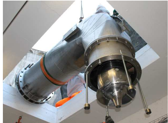
Figure 19 : The Diagonal turbine set at the foot of Montsalvens dam (CH) (© Mhylab)
