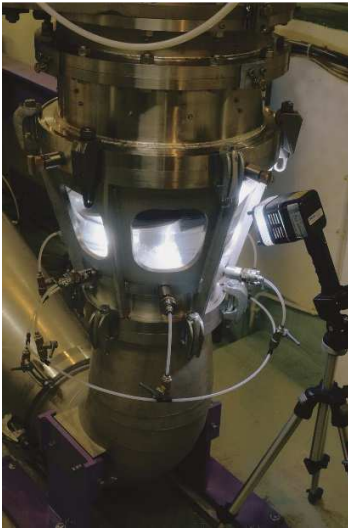
Figure 16 : Cavitation test on the S-shape Diagonal turbine (© Mhylab)
