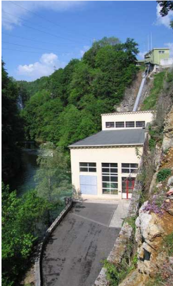
Figure 10 : Montcherand power plant where the test bench is set (© Mhylab)
